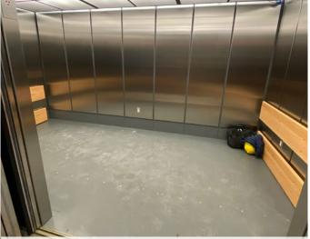
An elevator had to be constructed to accommodate the many staff members needed to accompany a heart surgery patient. In fact, two regular elevator shafts were combined into one cardiac unit.
