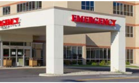
ORMC's existing Emergency Department entrance, which was completed in 2011
